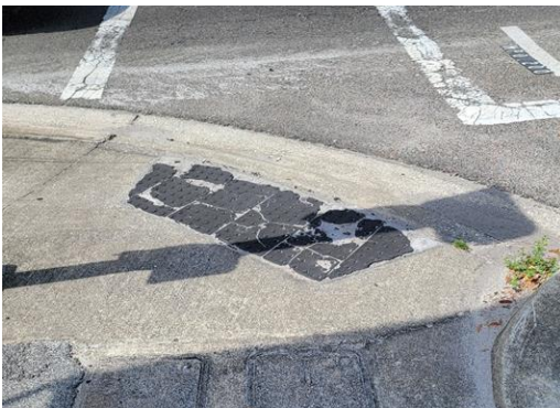
Figure I-3. Deteriorating accessibility feature, Corner of Orange Ave & Center St
