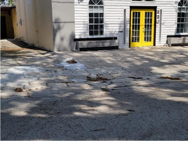
Figure I-30. Deteriorating Drive / Sidewalk, 220 Palmer
